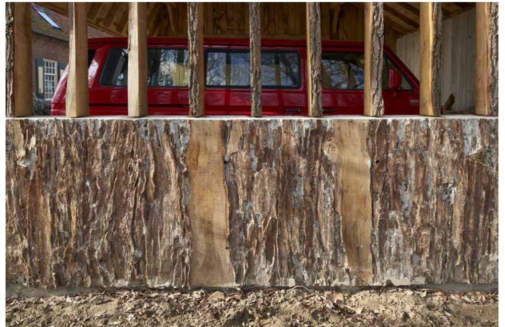
oak elements in cladding and roofing; iron traces in wood, woodprint in concrete and 'barked concrete,
