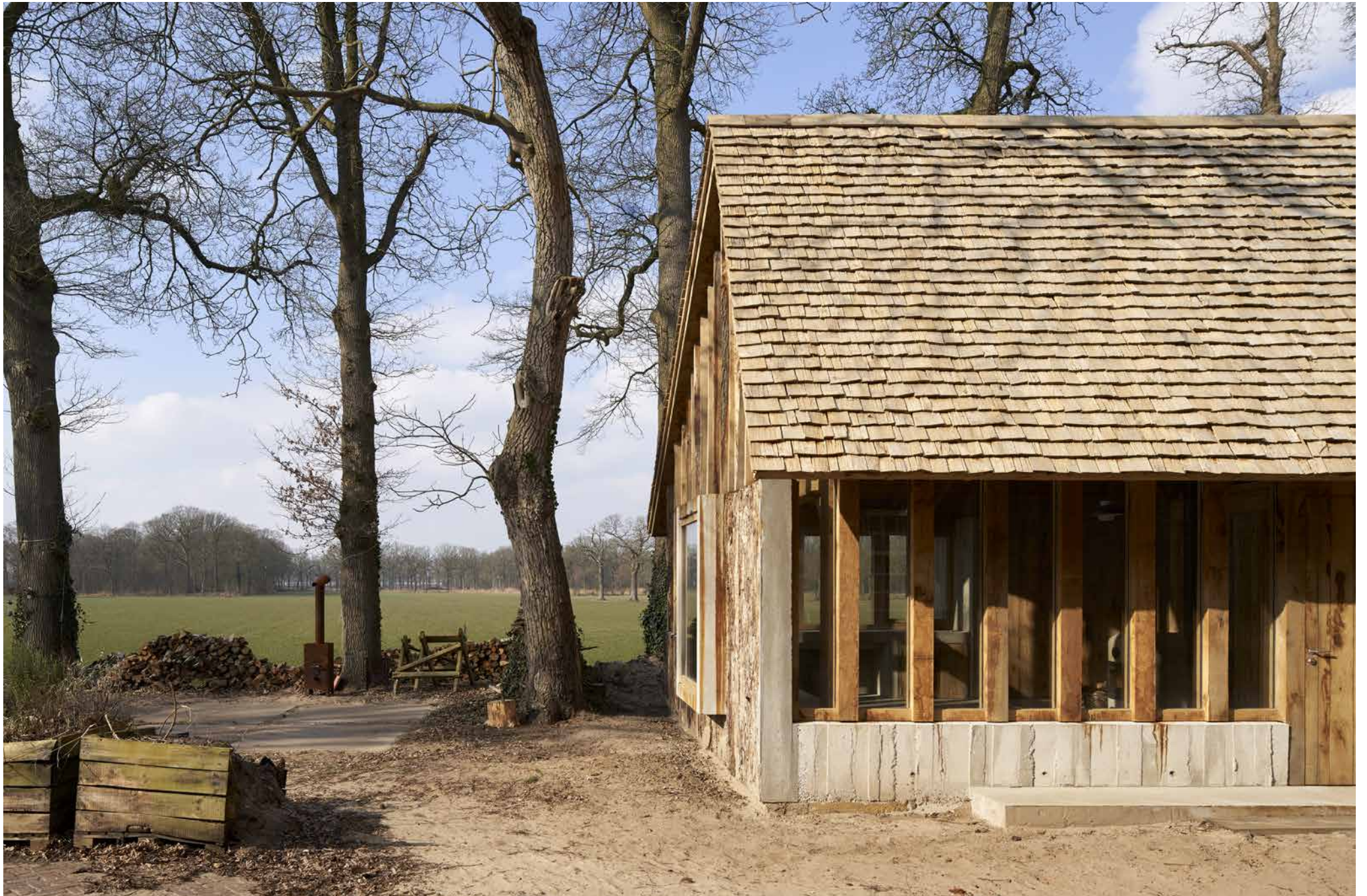
façade of workshop cum meeting room in oak, concrete and glass
