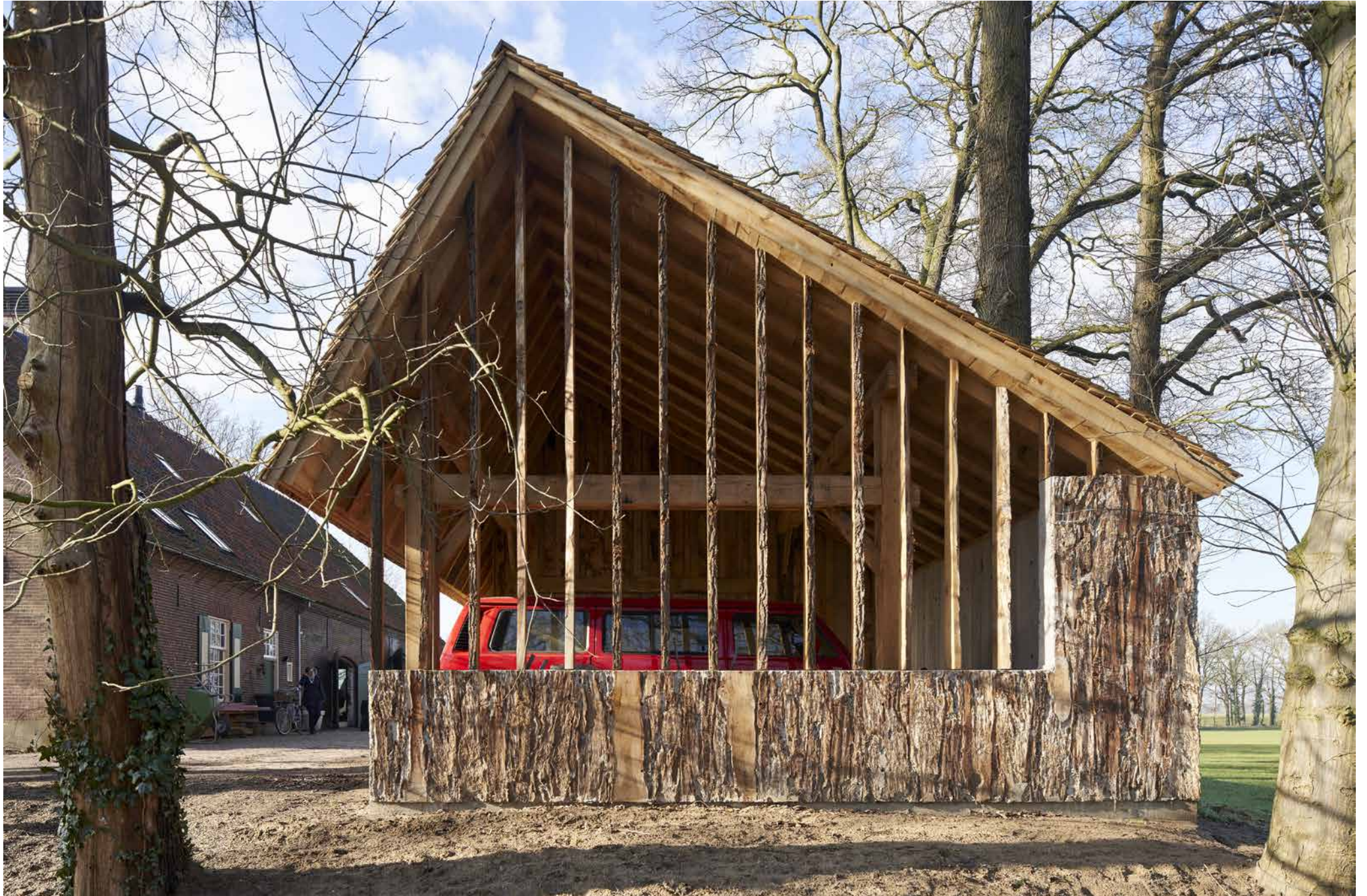
vertical slats create a diaphanous enclosure of the carport
