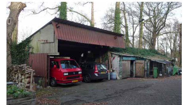
obsolete collage of shelters and sheds
