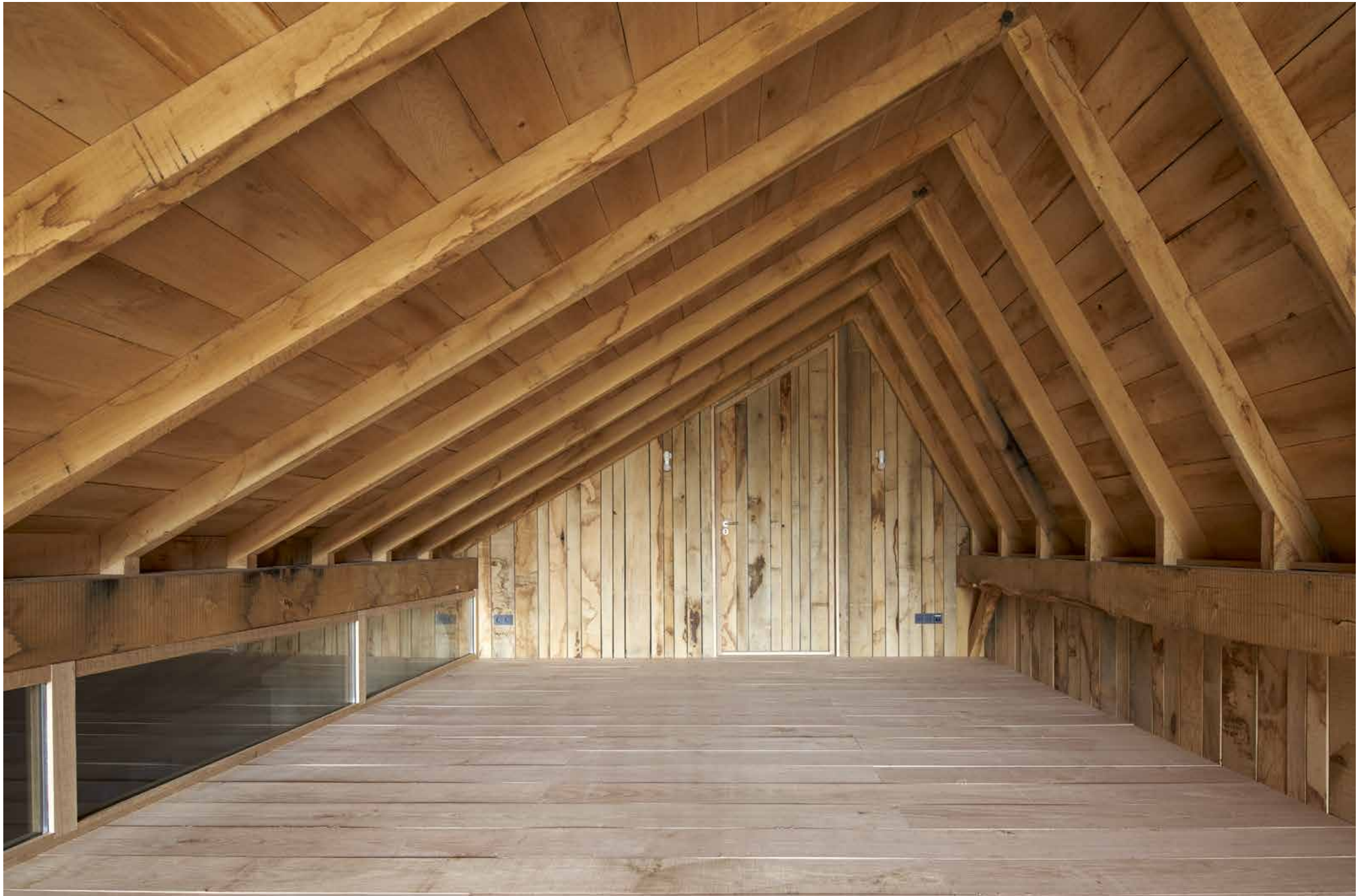
a glass slit in the loft floor allows daylight into the storeroom below
