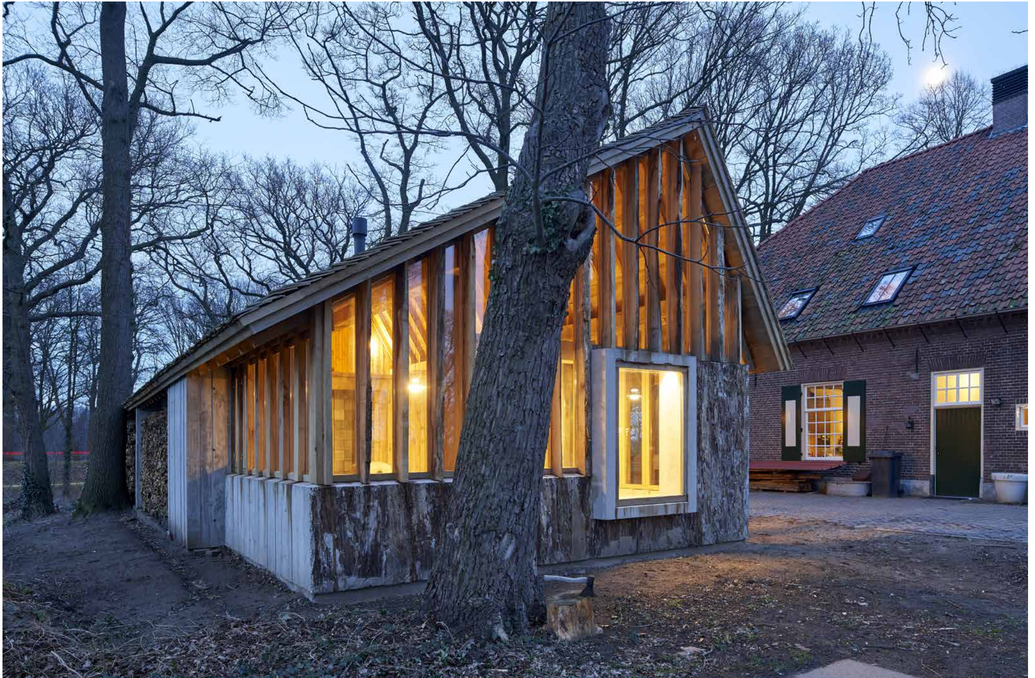
façade on field side has a gap in the foundation and roof to accommodate one of the existing oak trees; a subtle design accent
