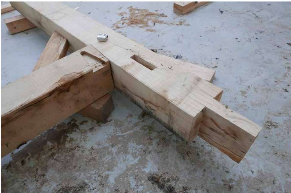
top: squared trunks - bottom: tiebar coupletruss
