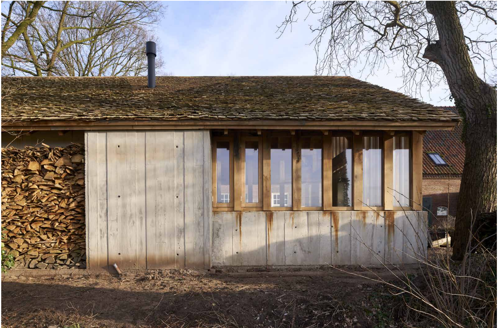
façade facing the fields with workshop on the right and firewood store on the left, tannic acid has left beautiful traces on the concrete
