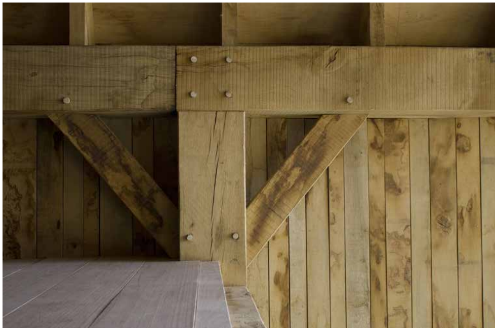
oak components in stringers, rafters, truss and wall
